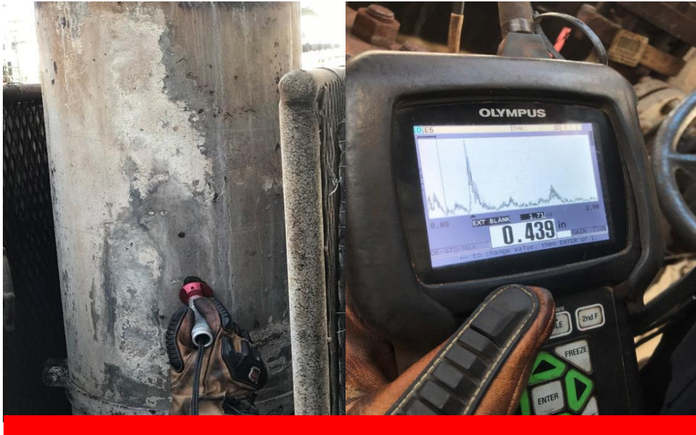
Fig. 1 (Left) Ionix HS582i probe in use at US Oil Refinery by a Mistras Inspector. Pipe temperature readings at time of this inspection were 582°F (305°C). (Right) The thickness measurements were able to be repeated several times with minimal cool down periods.
